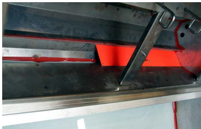
Fig. 3: First blank-off plate in a 2-fryer hood shown in final position. A second plate, needed to complete the installation, will overlap the first in the center of the hood.
