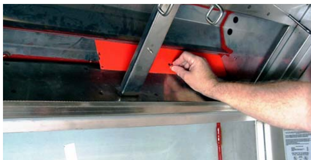
Fig. 2: Position a blank-off plate in the hood as shown and secure in place using its spring-loaded clip.
